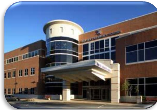
Goryeb Children's Hospital
